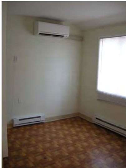
Interior Heat pump air handler
