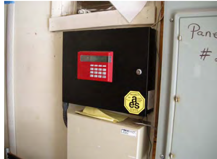
Fire alarm master panel
